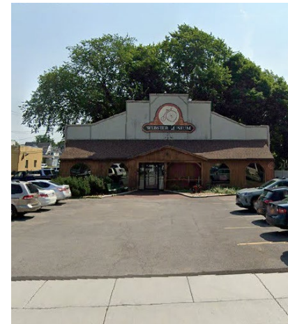
Webster Museum & Historical Society Climate Control and Façade Improvements
