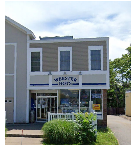
Webster Hots Walk-Up Window and Patio Upgrades
