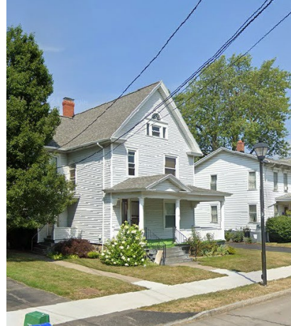
19 Lapham Park Porch Restoration
