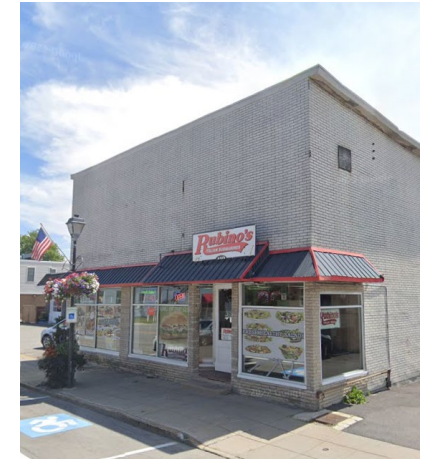
Rubino's Façade Restoration
