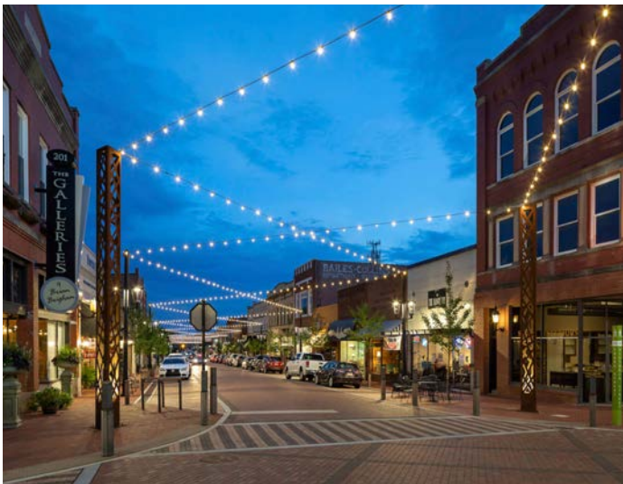
Trade Street in historic Greer, South Carolina is well-known for its iconic overhead lighting. A similar treatment is proposed for Main Street in Webster to enhance the quality of the space for events.
