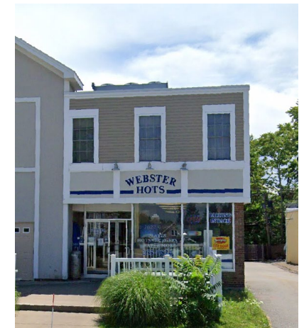
Webster Hots Walk-Up Window and Patio Upgrades
