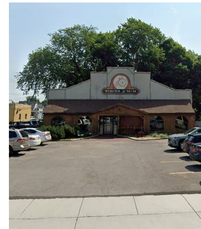
Webster Museum & Historical Society Climate Control and Façade Improvements
