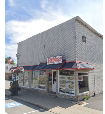
Rubino's Façade Restoration
