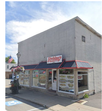
Rubino's Façade Restoration
