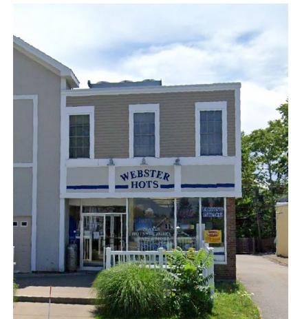
Webster Hots Walk-Up Window and Patio Upgrades
